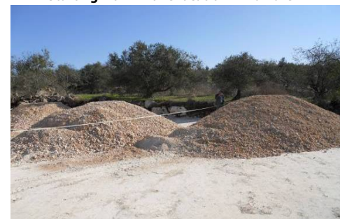
Starting work in another location in Tulkarem
