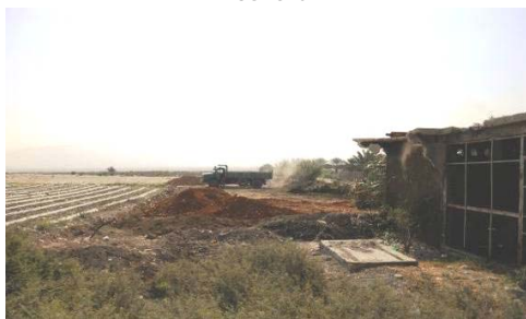
Starting work in one location in Jordan Valley
