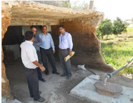
Field visit- one of the potential wells in Jenin
