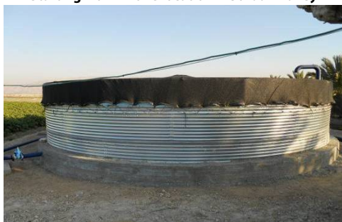
The above location after fabrication of reservoir in Jordan Valley
